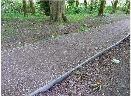
The pathway has been edged using thinner lumber to allow greater flexibility over the uneven terrain. It is held in place using 50mm x 50mm recycled plastic stakes cut to size on site.
