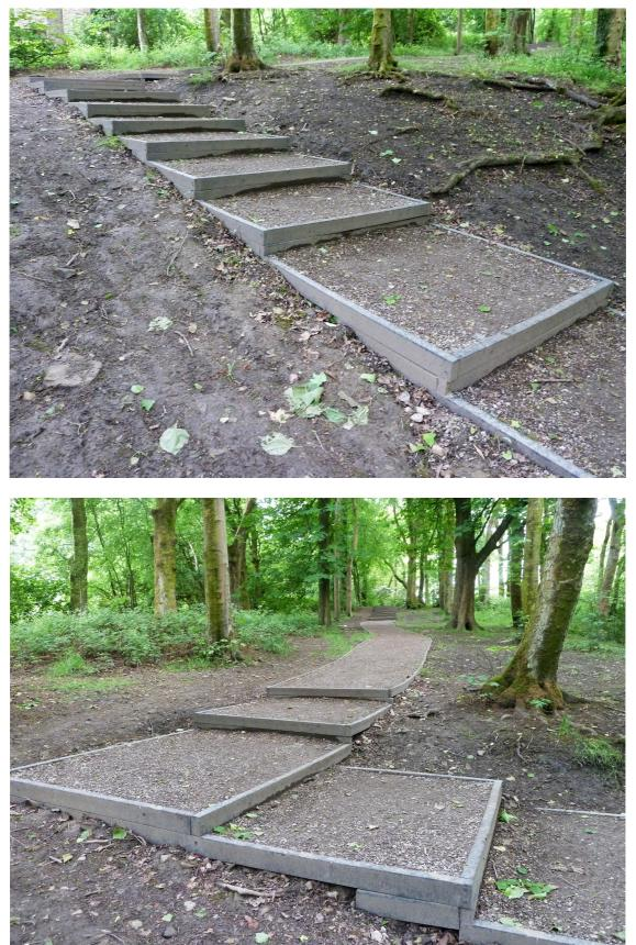
The steps have been constructed using thicker 50mm x 100mm to create a stable and long-lasting structure that will neither rot, split, splinter nor leach chemicals into this sensitive environment.
